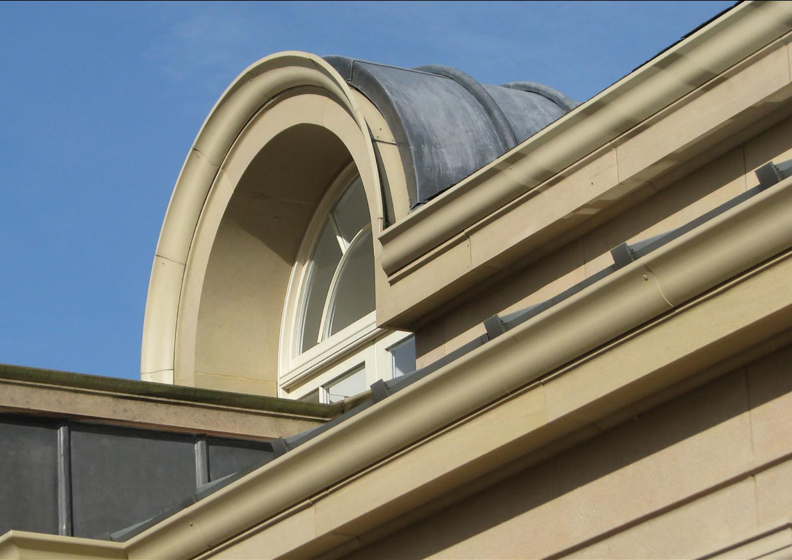
*Here is an example of stone effect finish gutter, designed to blend in with the brickwork of this prestigious property. Guttercrest matched and sourced the shade & finish from a small sample of the stonework.*
