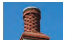
Private House, West Malling, Kent Parham Red Stock, I.SP.2 Spiral Brick to 600mm Diameter Column
